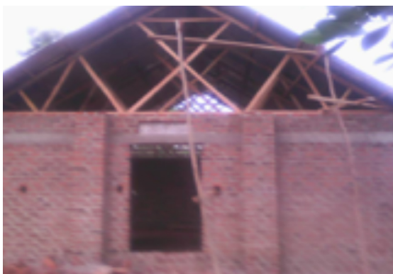
Uganda HQ before completion
